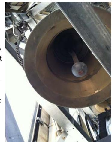
Swinging Bell—the clapper is in the middle and there are worn spots on the bell from where it hits the clapper when it swings. Also viewable is the big wheel with the metal chain, which is the mechanism that swings the bell.
